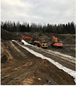
Mould for clay wall and drainage layers on<br/>both side it (Fortum).Construction on going in Sorsasalo summer<br/>of 2021 (Fortum).
